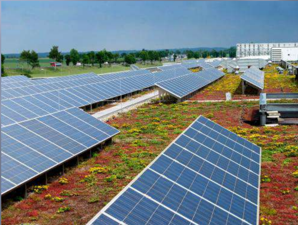
Blue-green roofs + pannelli solari
